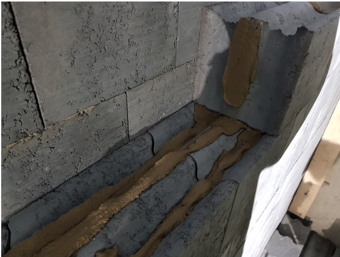
Image 1 Application of mortar (Note! It is not necessary to use mortar on vertical grooves)
